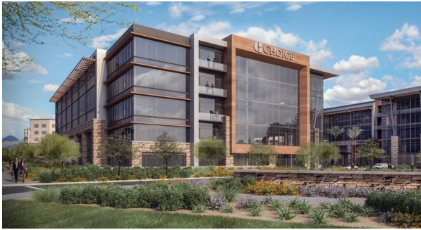
Cavasson Under Construction
