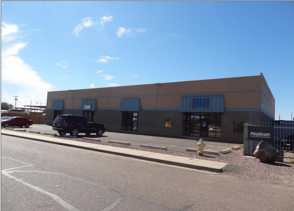
Front of Building
